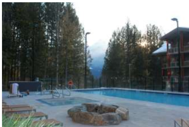
The new pool deck with outdoor, heated year-round pool and two additional hot tubs offers a private setting with mountain views at The Sutton Place Hotel – Revelstoke Mountain Resort
